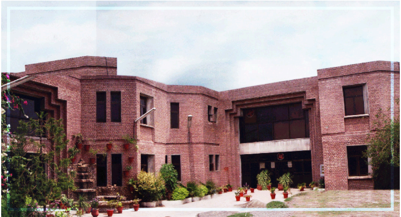
Figure 1 | REDO Eye Hospital, Rawalpindi, in Pakistan.
